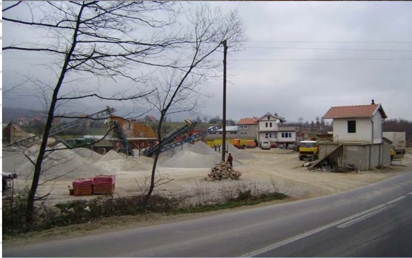
Aggregate screening plant near Hani i Llopushnikut
